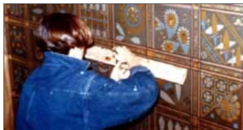
The task of preserving or restoring decorative work, such as the complex stencilling shown here, should only be undertaken by professionals who have specialized training. Photo: Alexis Elza.
