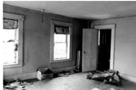
The interior of this 19th worker's house has not been properly maintained, but it may be as important historically as a richly ornamented interior. Its wide baseboards, flat window trim, and four-panel door should be carefully preserved in a rehabilitation project. Photo: NPS files.
