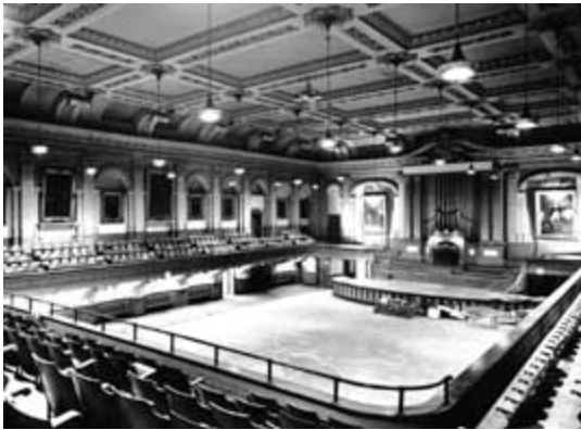
Many institutional buildings possess distinctive spaces or floor plans that are important in conveying the significance of the property. This grand hall, which occupies the entire floor of the building, could not be subdivided without destroying the integrity of the space. Photo: NPS files.
